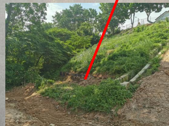
Toe slope sheet piles
