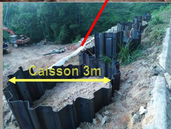
Caisson 3m piles at mid slope- 9m deep
