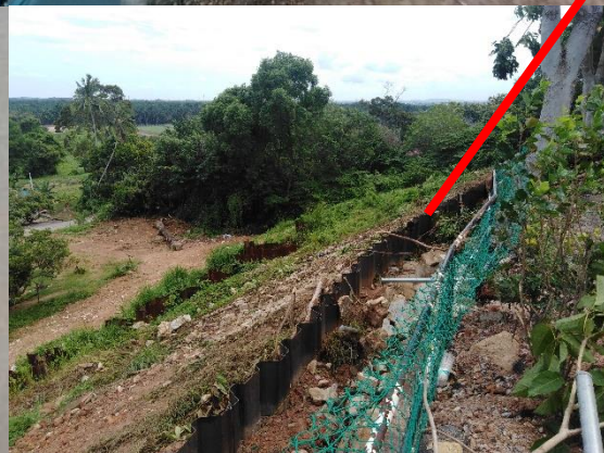
Crest slope sheet piles
